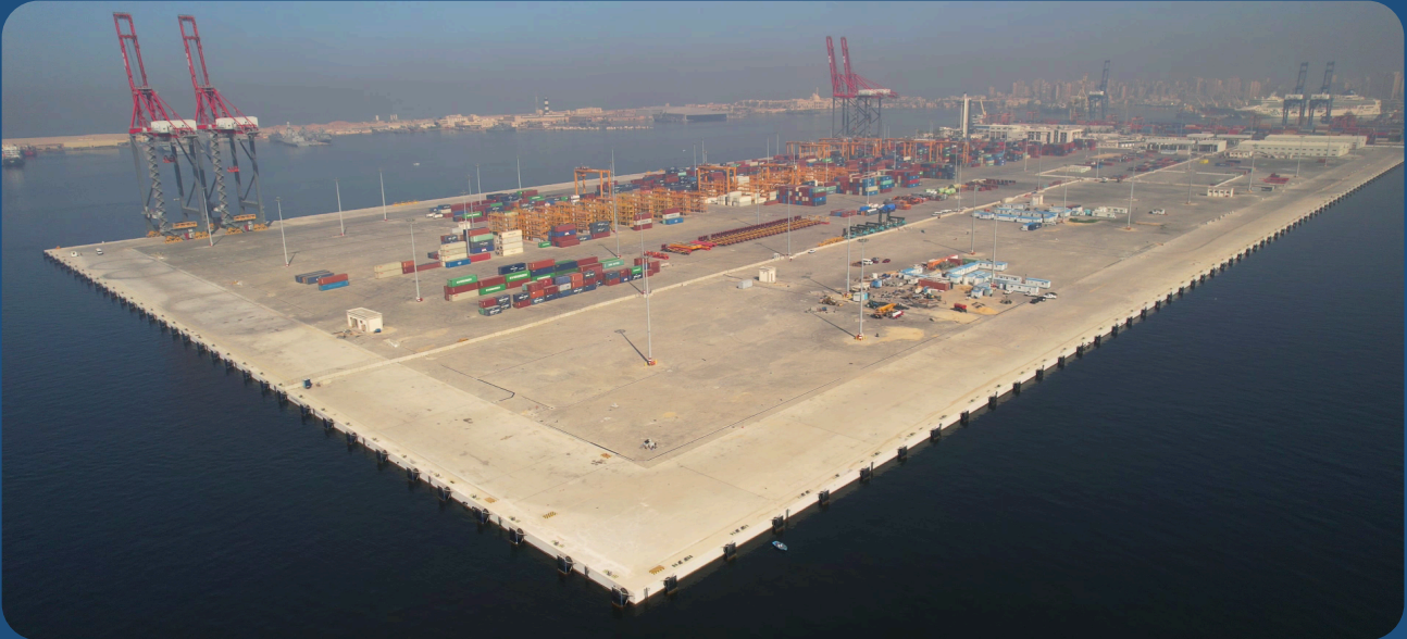
ALEXANDRIA TMT TAHYA MASR MULTI-PURPOSE PORT QUAIES 62-55
