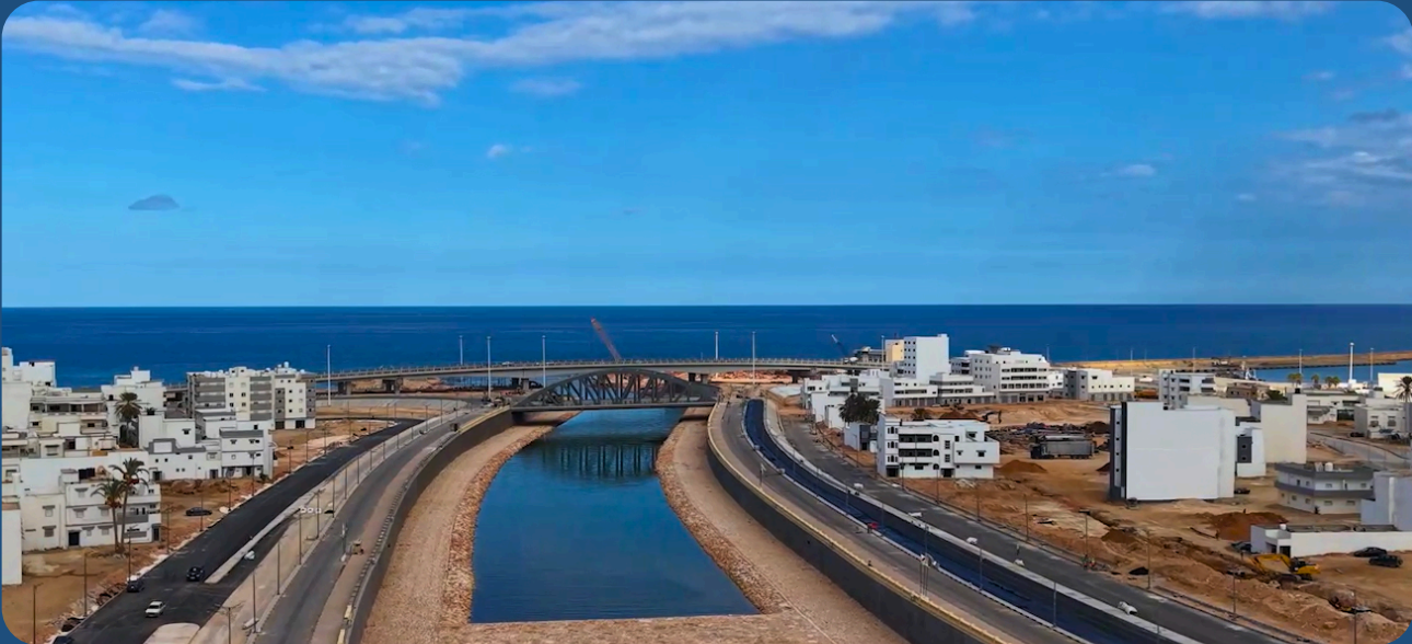
WADI DERNA, LIBYA CONSTRUCTION PROJECT FOR VEHICLE BRIDGE NO. 5 & 6
